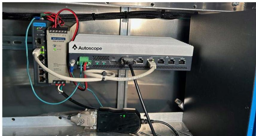
4. Connect the ground screw on the front of the processor and near the power connector on the PoE switch to earth ground.
